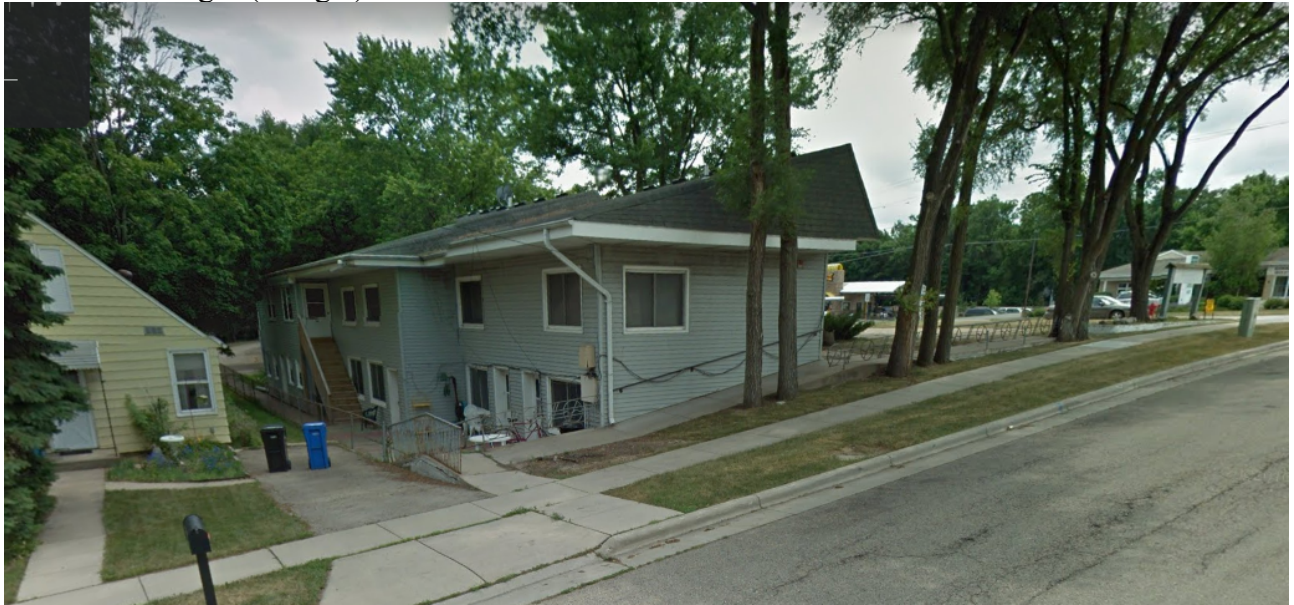
Figure 1 View from Northwest / Lakeview Ave showing and single-family residence. (July 2011)
