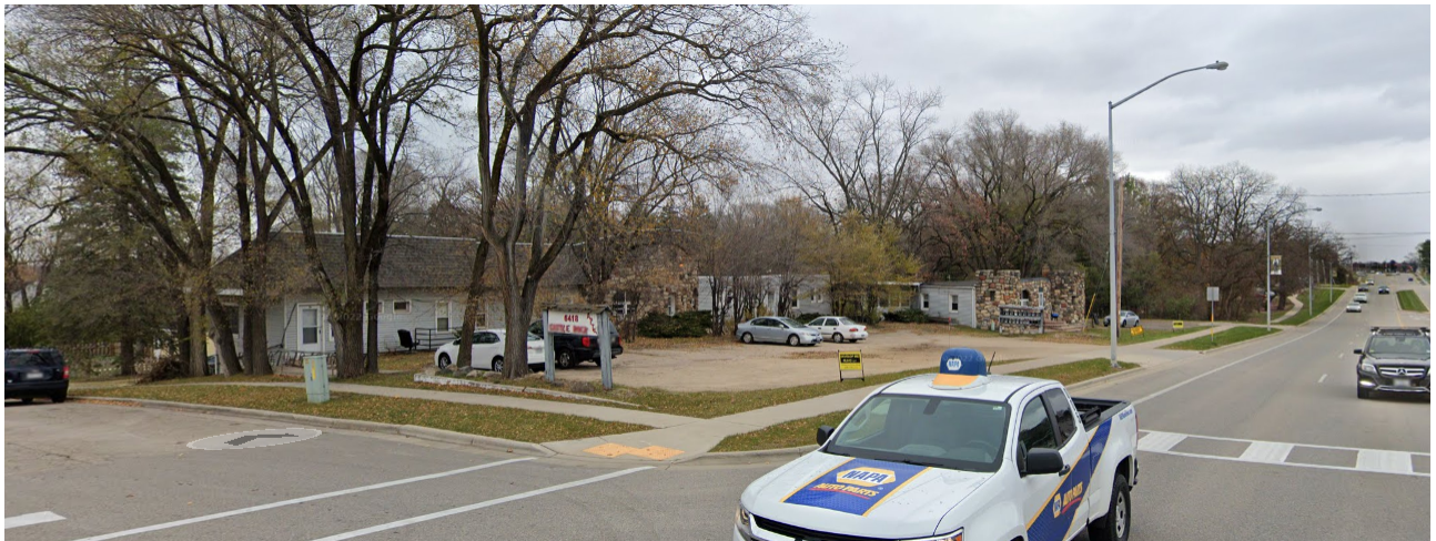
Figure 2 View from Southwest (November 2021)
